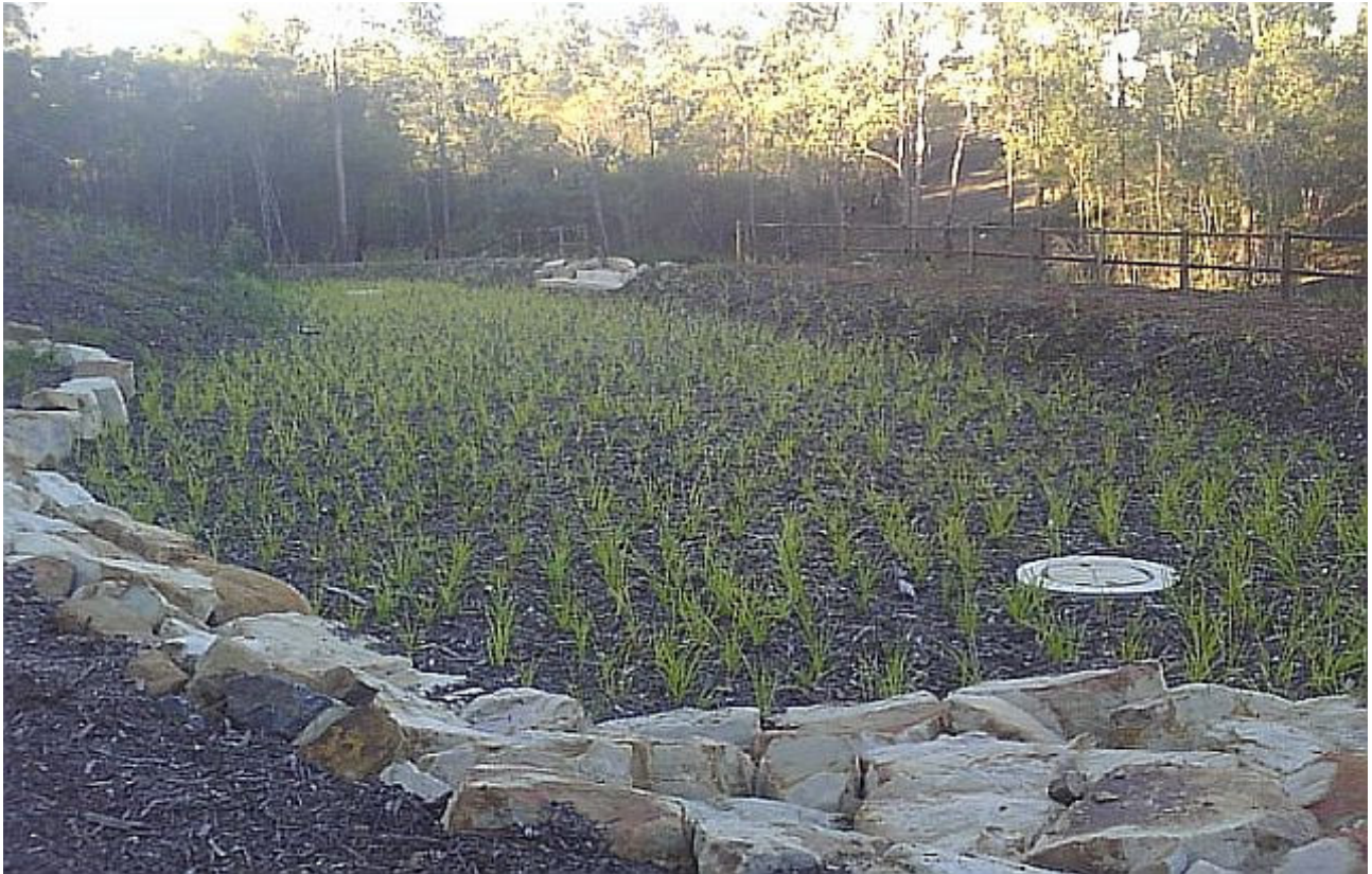
Figure 3-4 Water body Bioretention Pretreatment System
