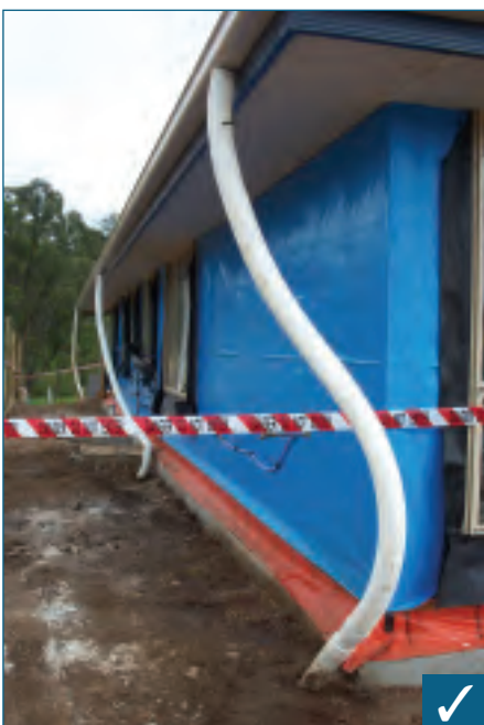
Temporary roof water connection
