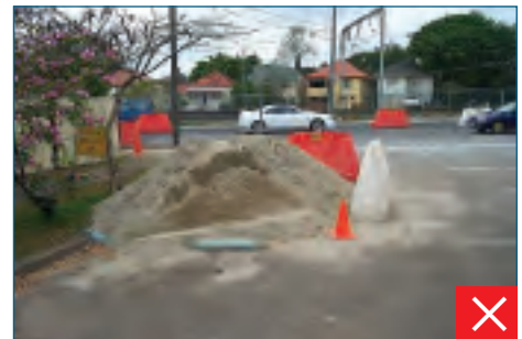
Don't store stockpiles on hard surfaces without suitable protection
