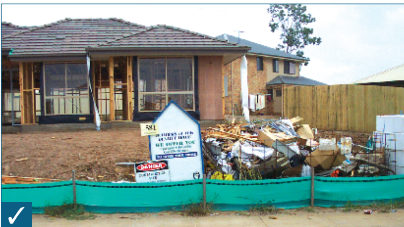
Sediment fence and best practice building site
