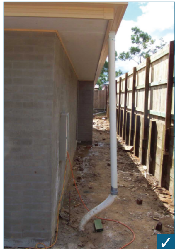
Temporary roof water connection
