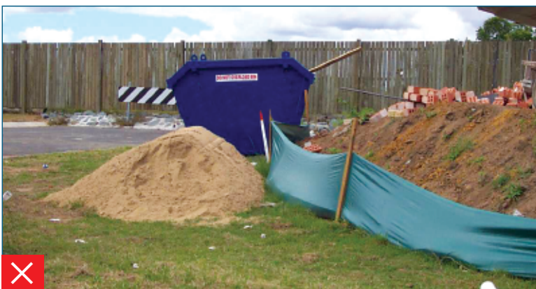
The stockpile must be located behind the sediment fence
